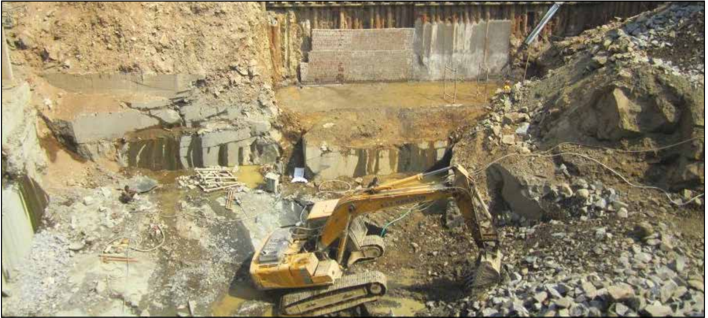
Excavation work with rock cutting activity on Site
