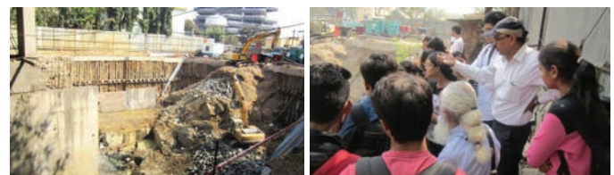
Site Visits , Inspection and Instructions.
