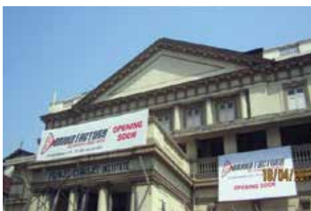
Gable end wall pediment
