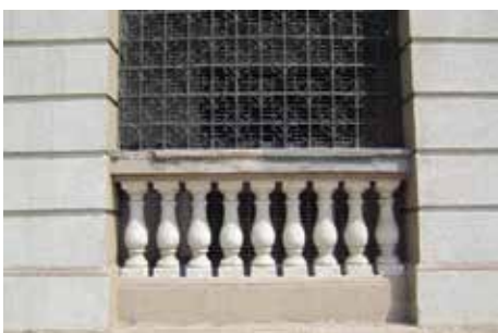
Baluster feature detail at the bottom of The semicircular arch.
