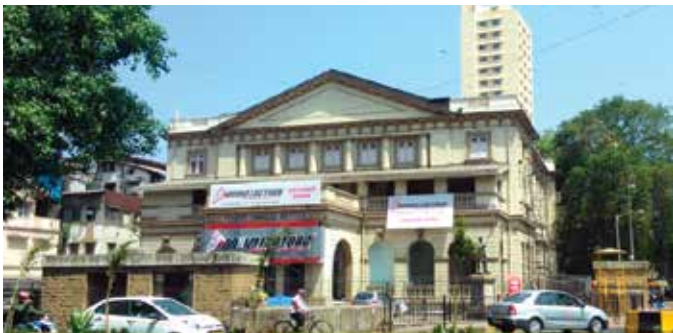
South façade and main entrance. The entrance view is blocked by recently constructed entrance of the subway.
