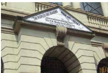
Key stone feature detail over the semicircular arch.
