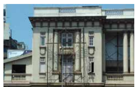
Doric style columns used as elevational Feature near window on the east façade.
